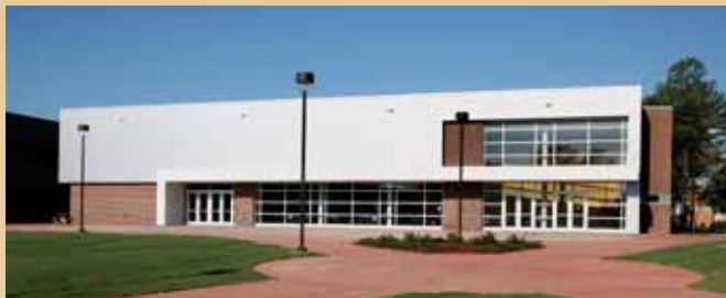
The new University Center Annex
