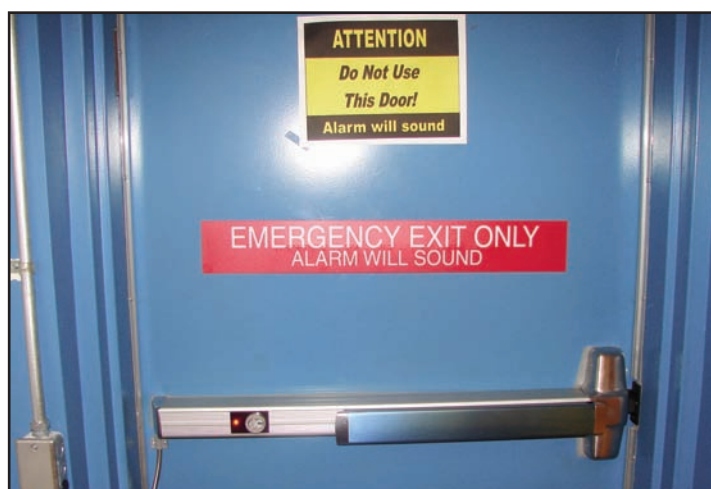
The new emergency alarms put in the residence halls over winter break were installed as a safety measure due to the Virginia Tech shootings April 16, 2007.
