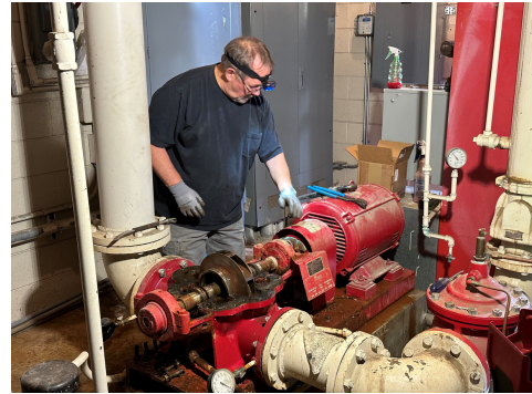
Library – fire pump repair
