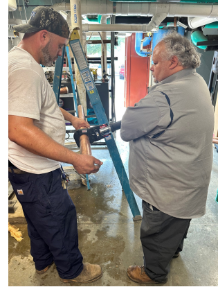
Pine Hall - water line repair
