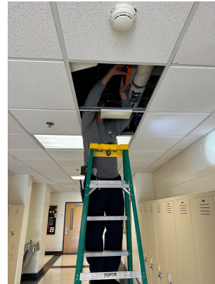
Moore Hall - hot water, actuator replacement
