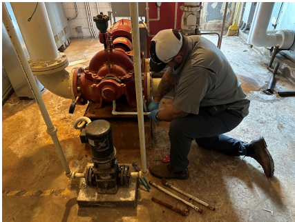
Library – fire pump repair
