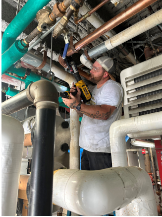
Pine Hall - water line repair
