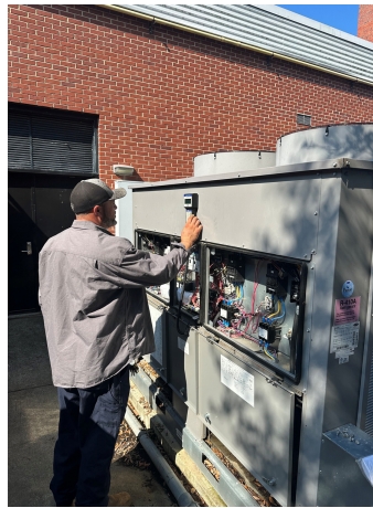
DF Lowery - chiller repair
